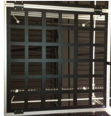
Ceiling panel installed in Gordon Grid system
