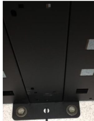
Post secured to slab floor
