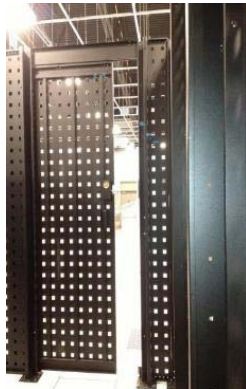
Internal door view
