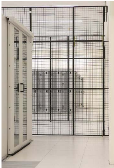
Welded wire barrier
