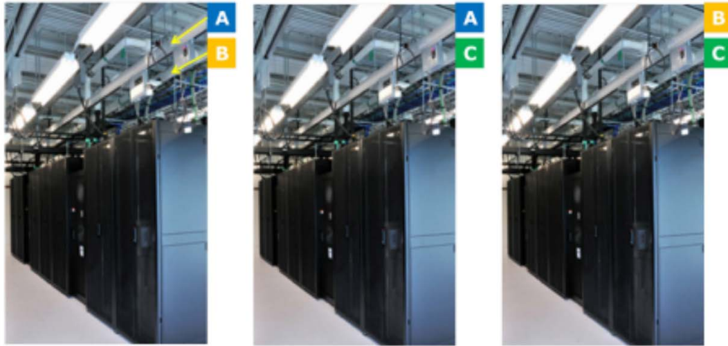
Power supplies to cabinets from bus bars from alternate UPS's
