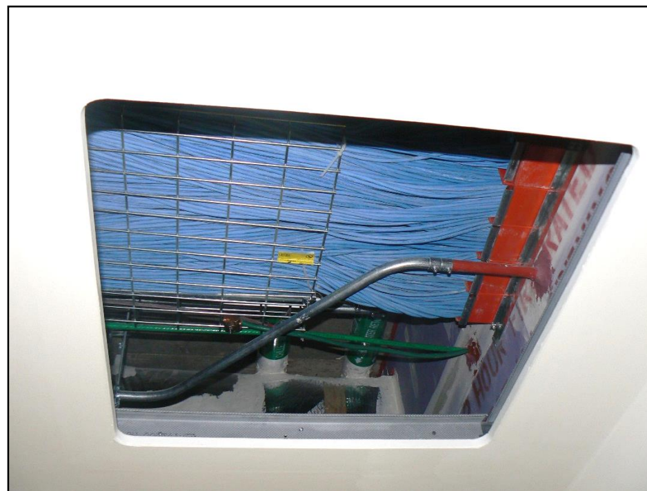
Above the ceiling
