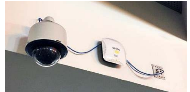
Photo taken at McCarran Airport in Las Vegas by our awesome marketing person – Anyone could jump up and pull out the patch cord to the surveillance camera and wireless access point.
