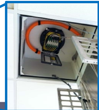
Exhibition Consolidation Point Zone Cabling
